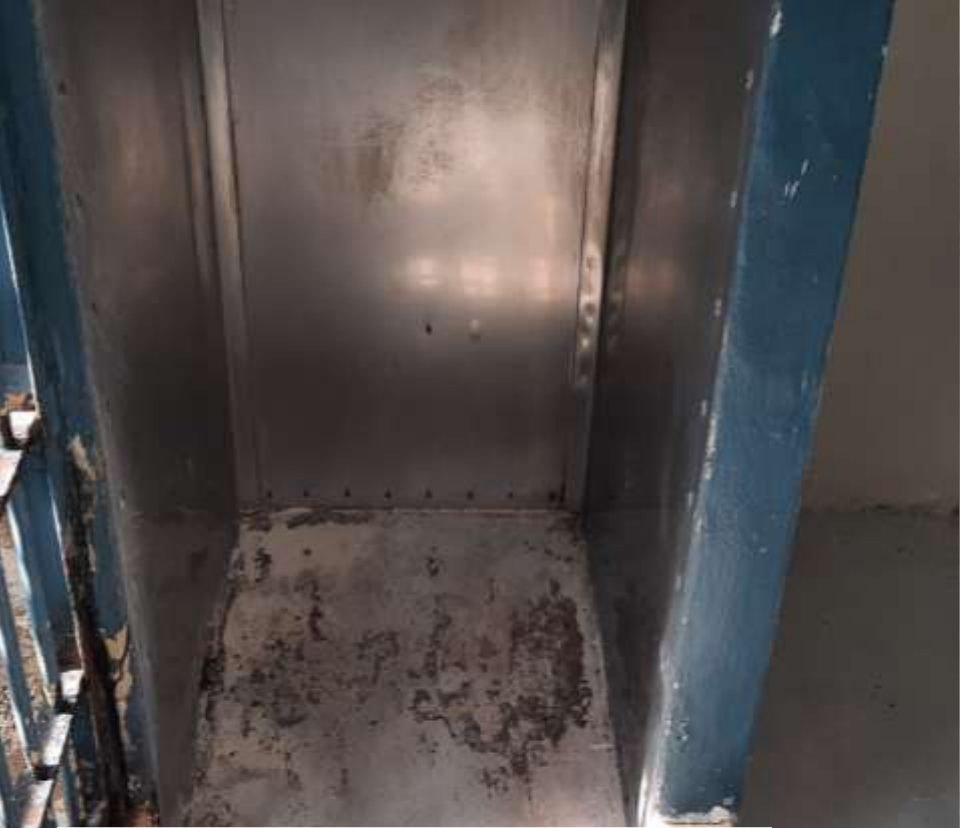
1975 Shower enclosure with Stainless Steel Insert
